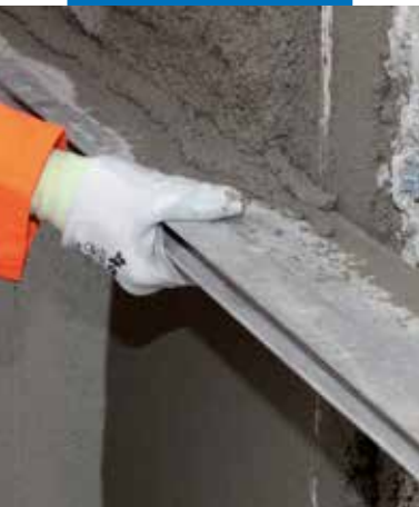
Levelling off Mapegrout 430 with a straight edge
