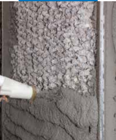
Application of Mapegrout 430 by spray
