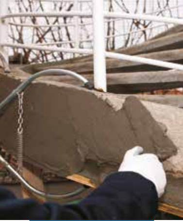
Application of Mapegrout 430 by trowel
