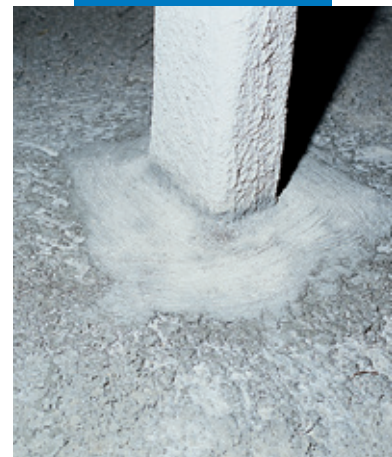
Pillar waterproofed with Idrosilex
