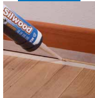
Filling the joint
