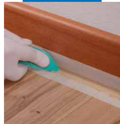
Finishing off the surface
