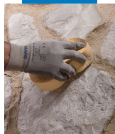
Finishing the surface with a sponge
