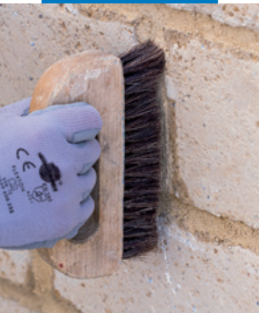
Finishing the mortar joints
