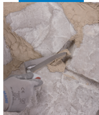
Pointing the joint in a stone wall
