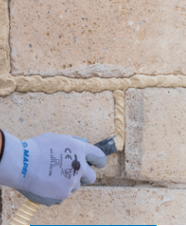
Removing the excess mortar
