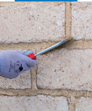
Cleaning the mortar joints with a millet brush
