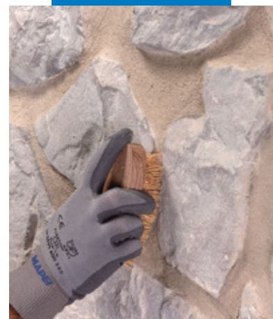
Finishing the surface with a millet brush
